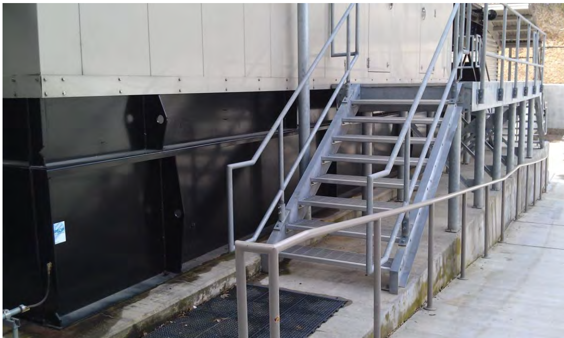
Figure 2: Diesel Fuel Tanks below the Generators
