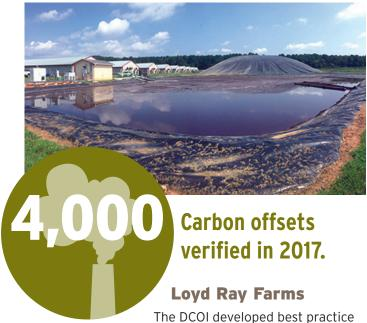
guidance for swine farmers from six years of experience managing and conducting research at the swine-waste-to-energy system at Loyd Ray Farms in Yadkinville, NC. This system generates carbon offsets and Renewable Energy Certificates (RECs) by capturing the biogas that results from the decomposition of hog waste and using it to generate electricity on-site.
